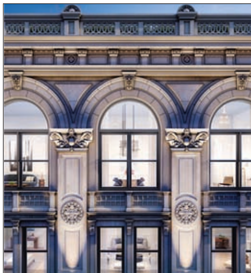
108 LEONARD- A dramatic 19th century Italian Renaissance Revival façade graces the building
