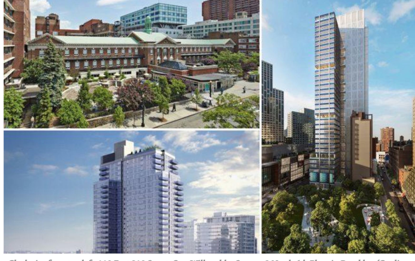
Clockwise from top left: 110 East 210 Street, One Willoughby Square, 2 North 6th Place in Brooklyn (Credit: Montefiore Health System and DBOX)
